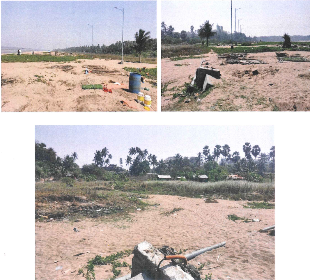
Figure 2 Erosion at Aksa beach and falling of the electric poles due to erosion.
